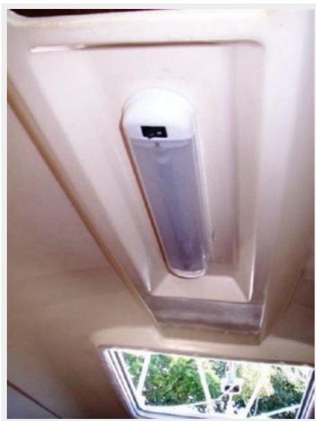
LED Light & Deck Hatch
