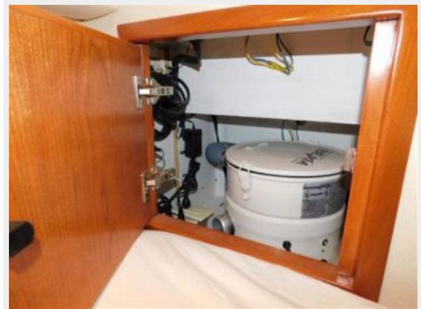
Charisma - VIP stateroom with central vac access compartment
