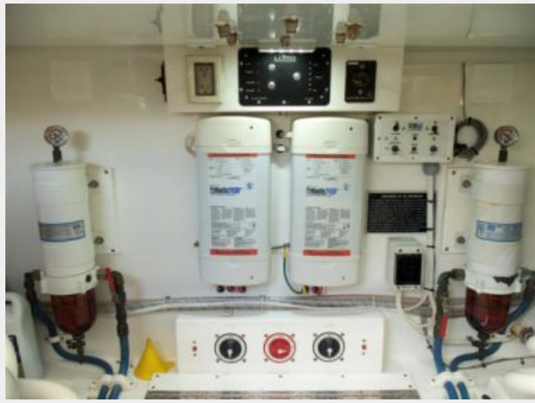
Engine Room Forward
