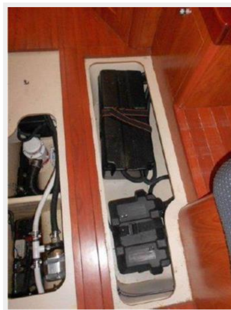
A view into the bilge (left) and battery compartment
