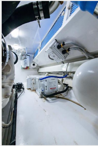
Paved For_Engine Room13
