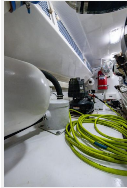
Paved For_Engine Room14
