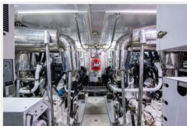
Engine Room Forward
