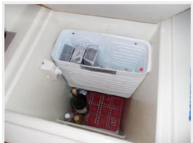
Refrigerator w Cold Plate
