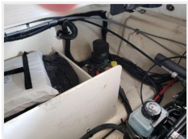
Engine Room Components
