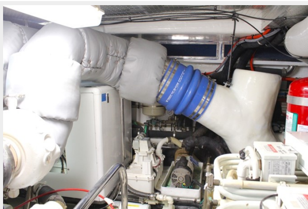
Engine Room Starboard 2
