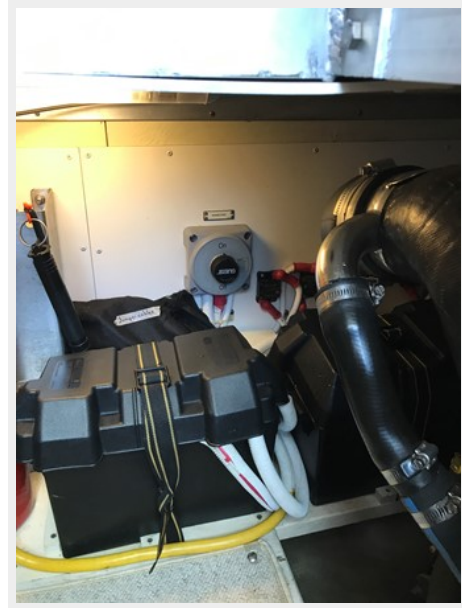
360 Carver SS - Engine Room
