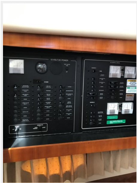
360 Carver SS - Distribution Panel
