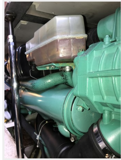
360 Carver SS - Engine Room
