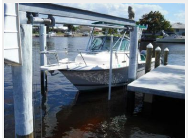
Lowered and in The Water
