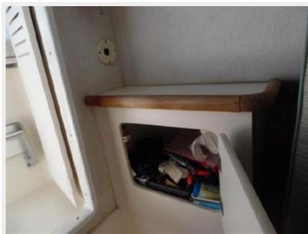
Interior Storage to Port
