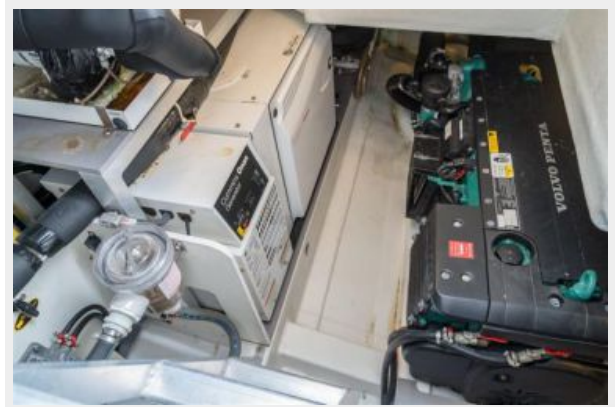
Engine Room Access
