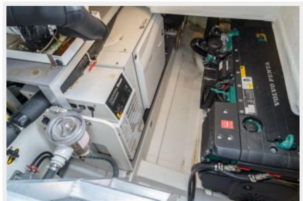
Engine Room Access
