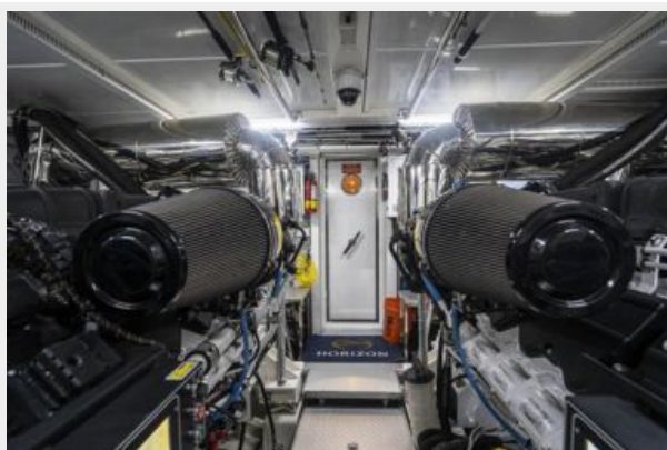
Engine Room Aft
