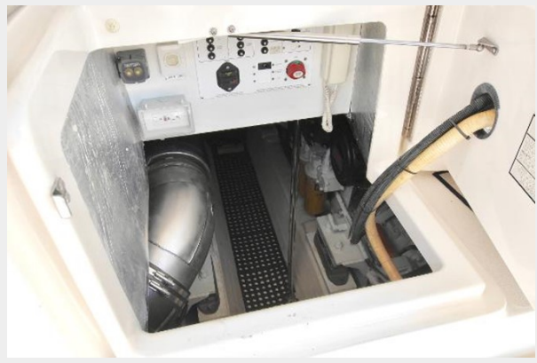
Engine Room Access
