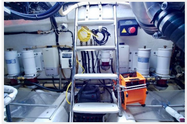
Steps into Engine Room
