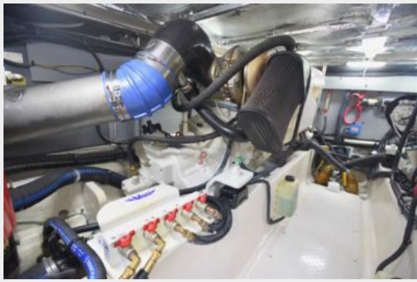
2004 Sea Ray 48 Sedan Bridge - Engine Room
