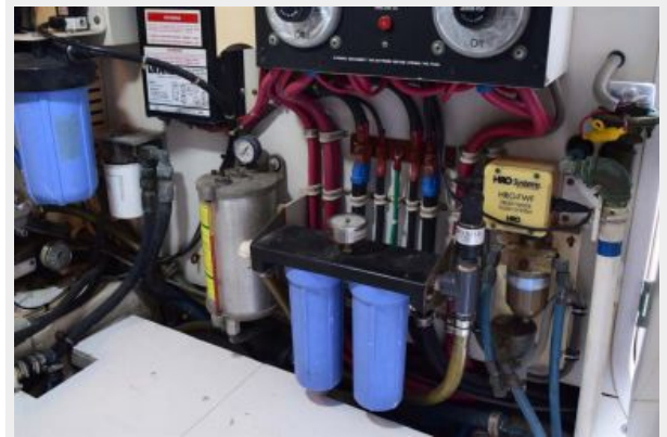
Fresh Water Flush System
