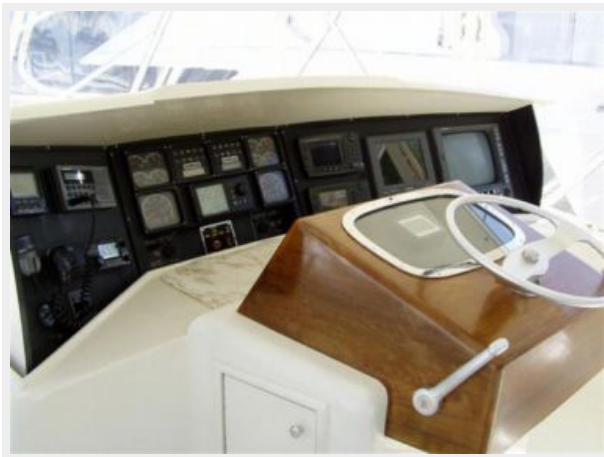
Flybridge Helm Electronics
