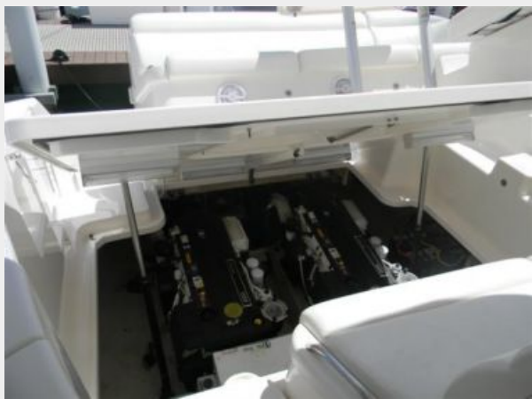
Engine Room Access
