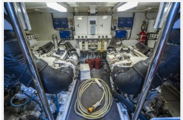
Rear Full Beam Engine Room
