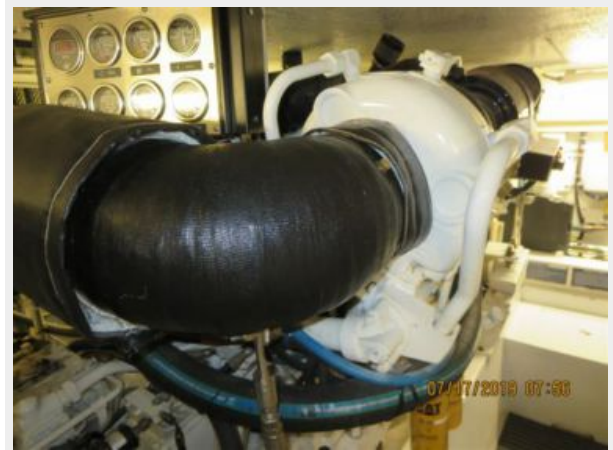
Engine room- new risers on main engines installed 7/19
