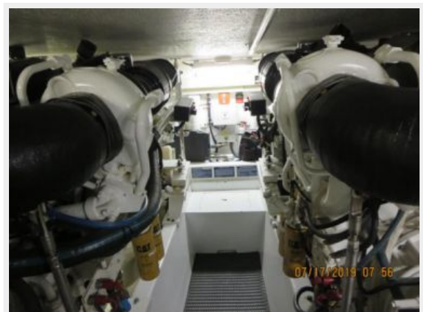
2002 60' Hatteras Convertible Engine Room
