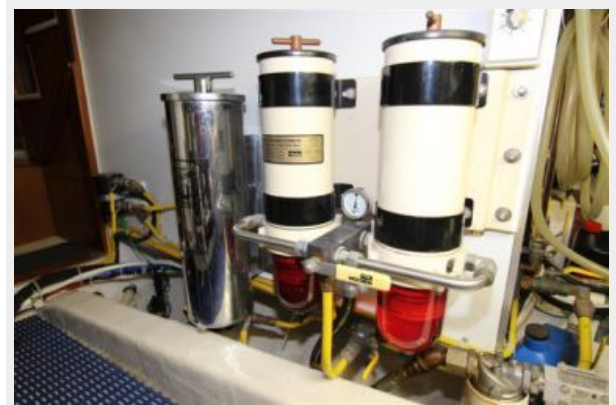
Starboard Dual Racor and Fuel Polisher
