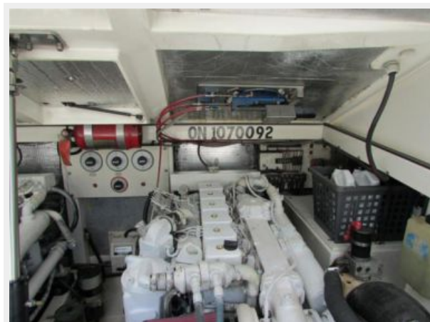
1998 Cabo 31 Express - Engine Room
