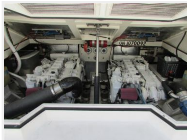
1998 Cabo 31 Express - Engine Room
