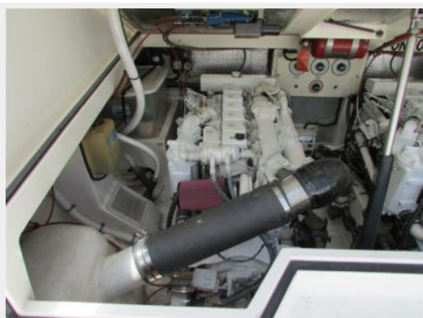
1998 Cabo 31 Express - Engine Room
