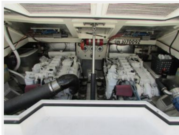
1998 Cabo 31 Express - Engine Room
