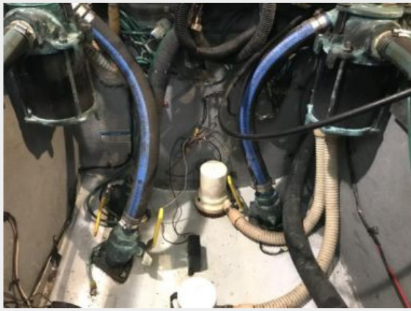
dry and clean bilge
