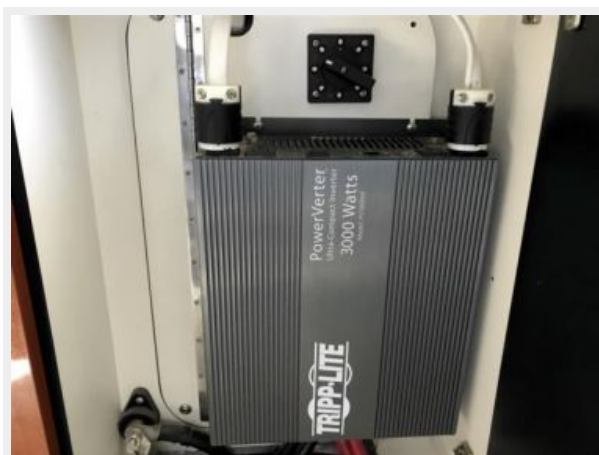
Tripp-Lite 3KW inverter
