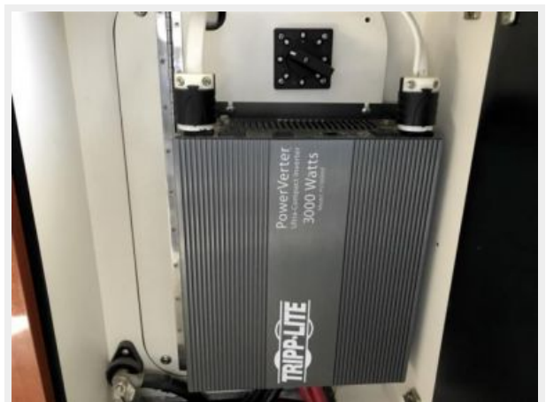
Tripp-Lite 3KW inverter
