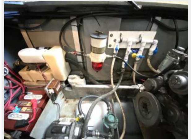
clean and organized engine room
