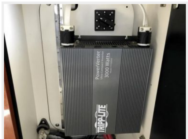
Tripp-Lite 3KW inverter
