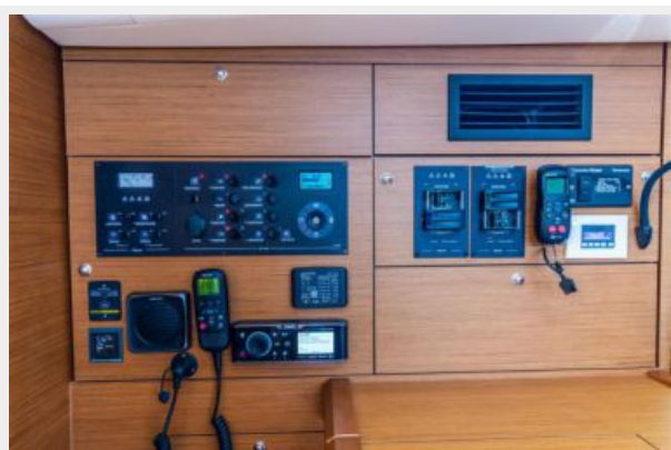
Main Distribution Panel
