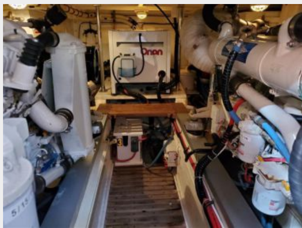
Twin Cummins engines, Onan generator
