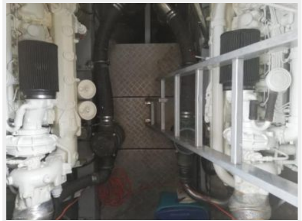
Engine Room Ladder Access
