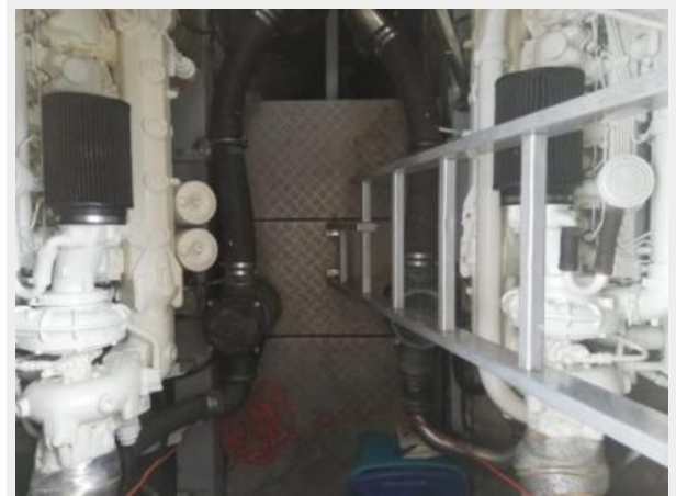
Engine Room Ladder Access
