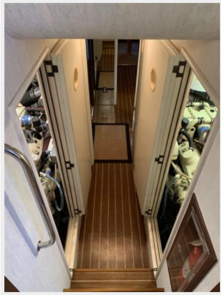
Hallway to Engine Room
