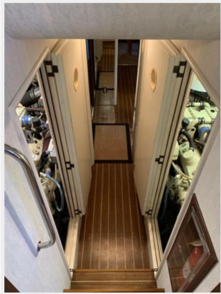
Hallway to Engine Room
