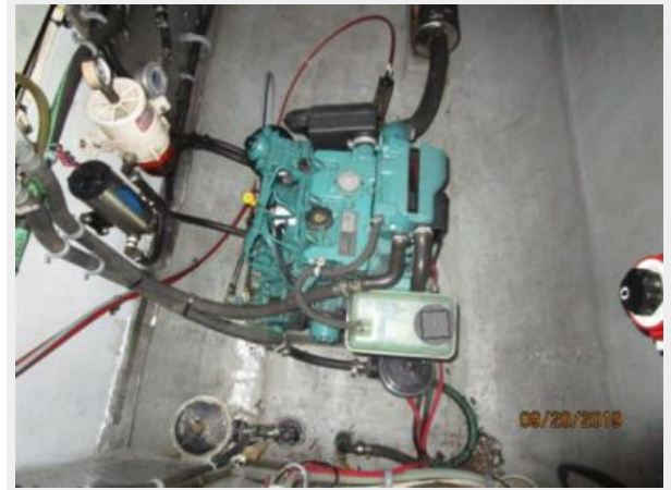
52 Zep Tepi port engine room1 9-20-19
