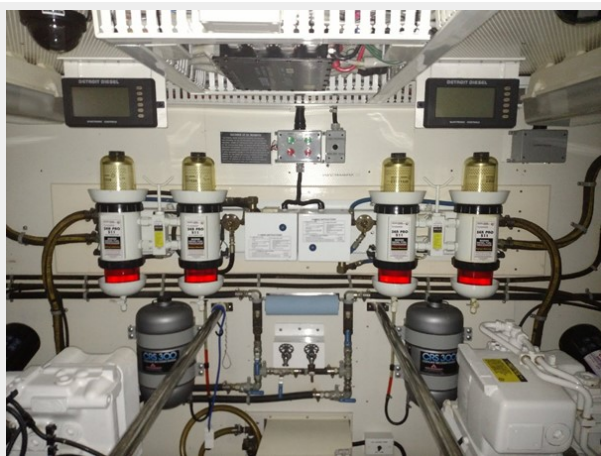
Engine Room Forward
