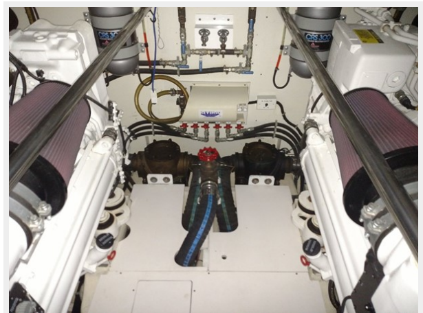
Engine Room Forward
