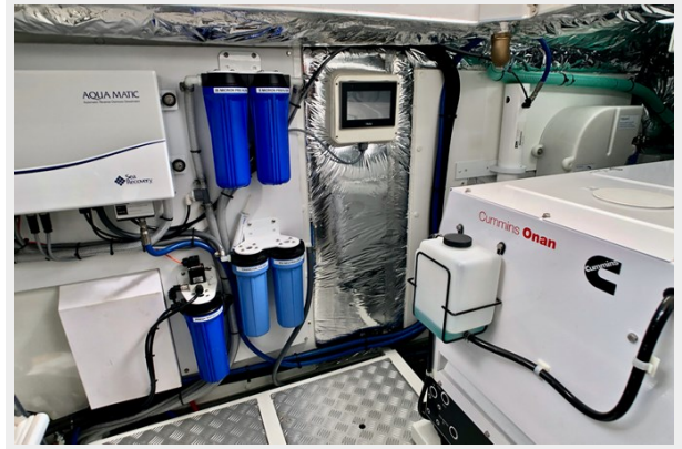
2019 Princess 70 Flybridge Engine Room
