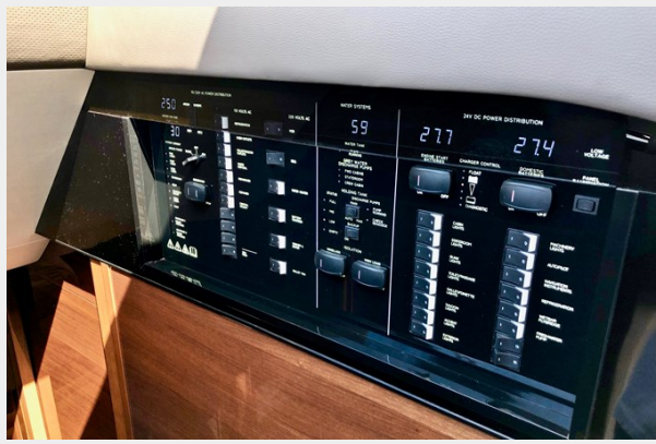
2019 Princess 70 Flybridge Breaker Panel
