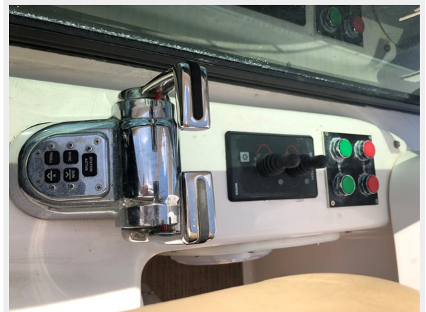
Portside Flybridge Wing Station
