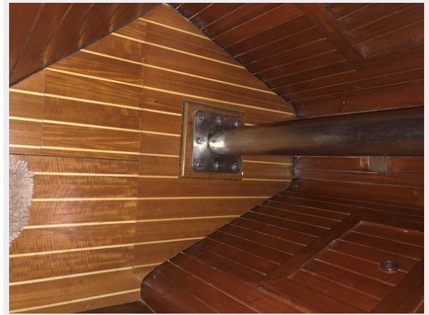
New cabin sole and compression post footing
