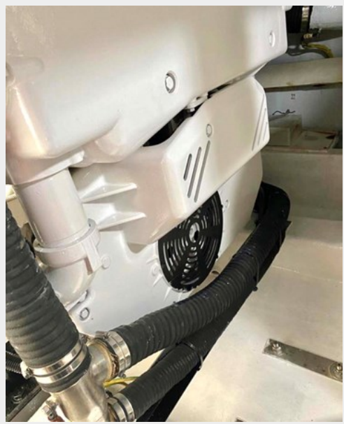
Engine Room Full Detail 2022
