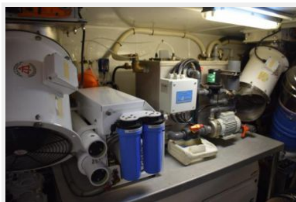
Watermaker - Hamman, Delta T ventilation
