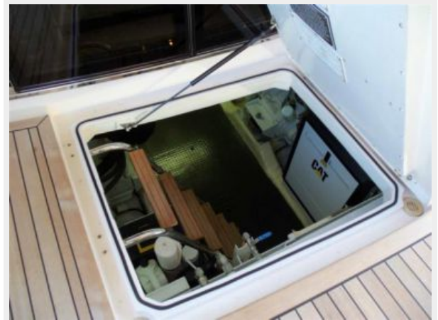
Engine Room Access
