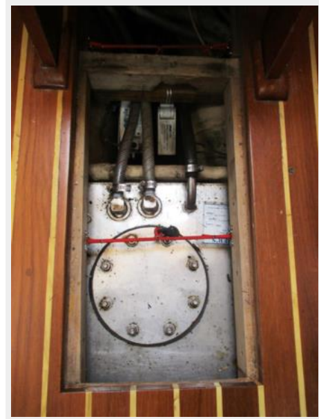
New water tank
