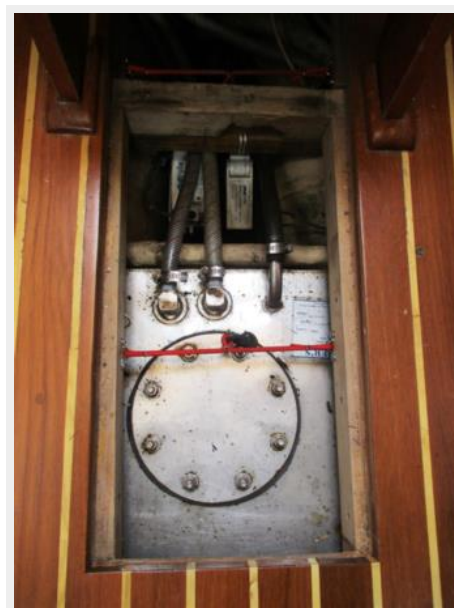
New water tank
