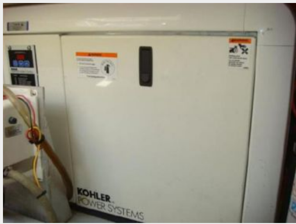
309 Generator Sound Shield
