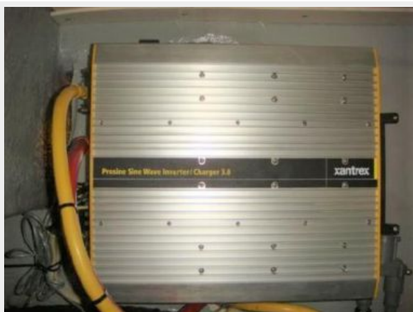
313 Xantrex Prosine Inverter
