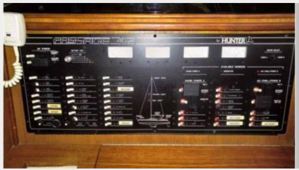
ELECTRIC PANEL AT NAV STATION
