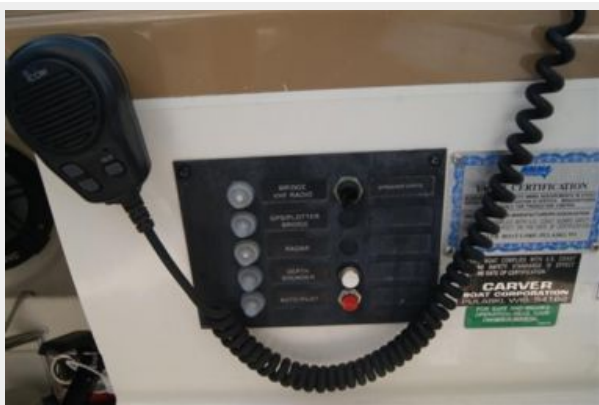
318 Bridge 12v Breakers
