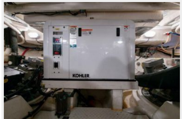
15_Engine Room 4, Generator
