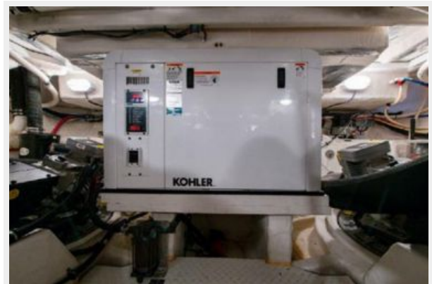
15_Engine Room 4, Generator
